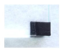
11. Put the glass in the channel. The dead end is shown at left, and the live end is shown at right.
