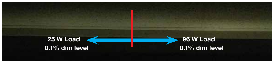
Figure 2: Cove Lighting After the Use of the Field Adjustment Knob Eliminates Mismatch without Costly Re-wiring
